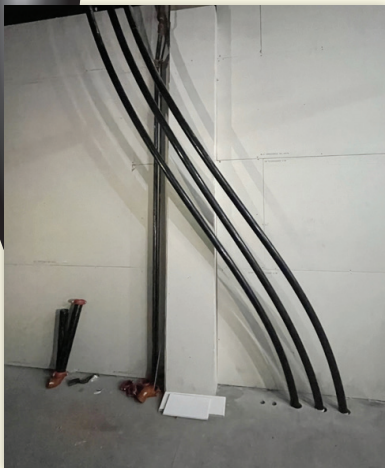
First Floor 2" DoubleTrac® piping around column.
