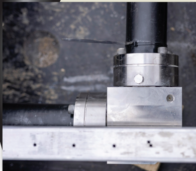
2" DoubleTrac® Double Containment 90° Elbow Fitting
