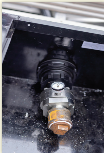
2" DoubleTrac® End Fitting terminated in steel UDC.
