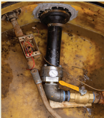
2" DoubleTrac® installed in existing underground transition sump.
